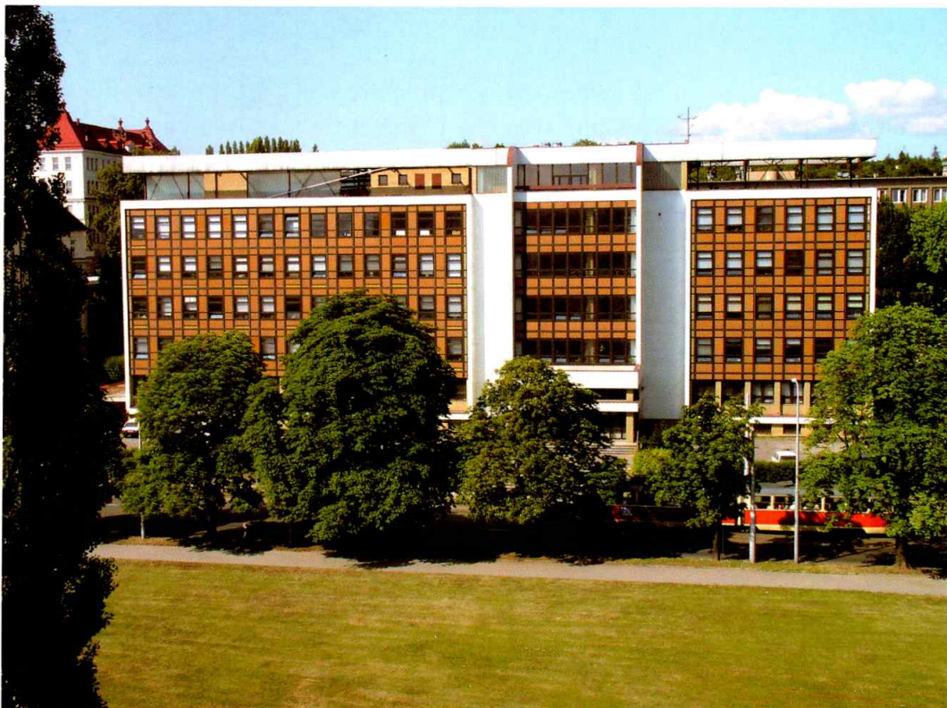
The building of the Institute of Analytical Chemistry in Brno.
